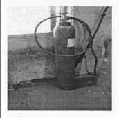
Fire extinguishers periodical checking (inspection and refilling ) not done in distillery area
